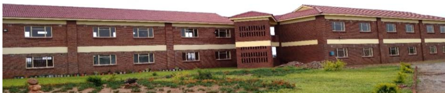
1. und 2. Bauabschnitt Mary Ward High School in Mbizo-Kwekwe
